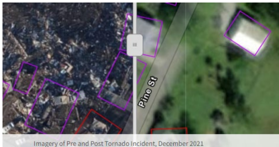
Imagery of Pre and Post Tornado Incident, December 2021
